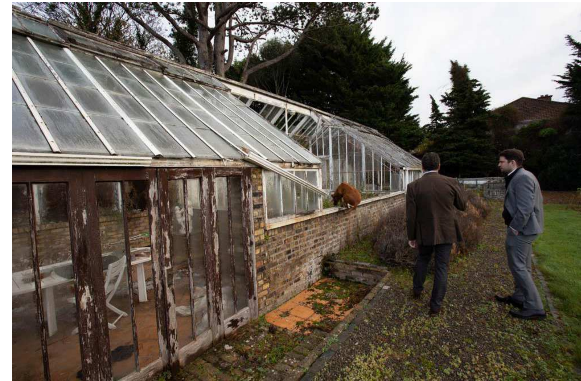
EXISTING Image showing the current condition of Vinery structure.
